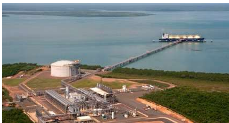
The Darwin LNG plant in northern Australia. (ConocoPhillips)
